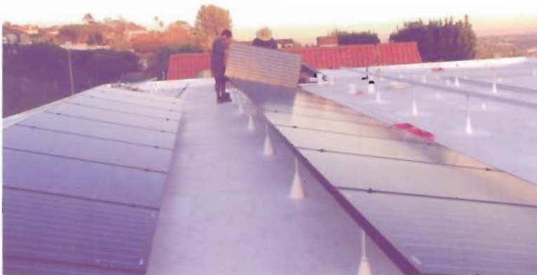
Installing the 64 solar panels in November 2009
