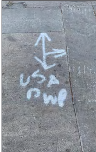
USA (UNDERGROUND SERVICE ALERT) AND DWP (DEPARTMENT OF WATER AND POWER)
