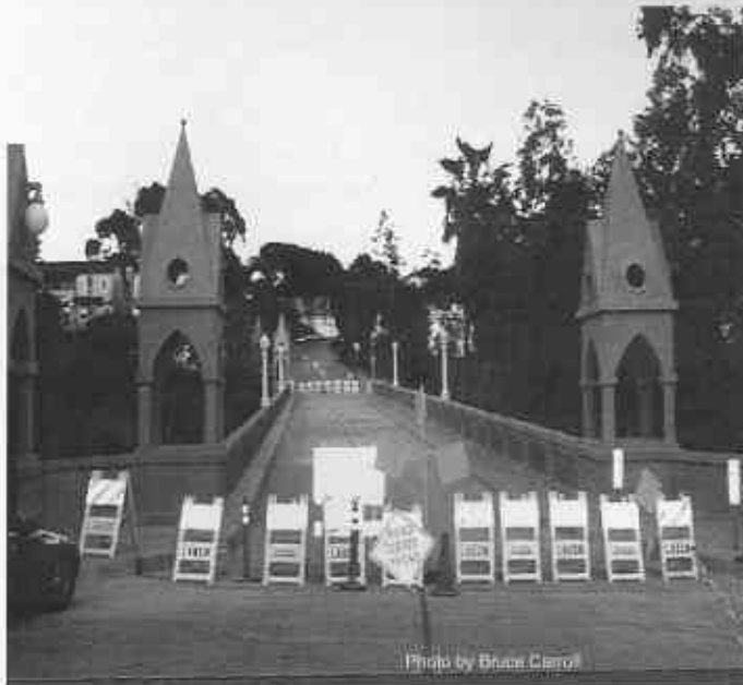
The Last Lonely Night for the Shakespeare Bridge April 18, 1998
