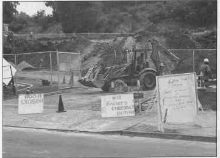
Since these signs were drawn, Barnsdall Art Park Museum employees have reportedly agreed not to dig tunnels if MetroRail construction workers won't make anymore signs.
