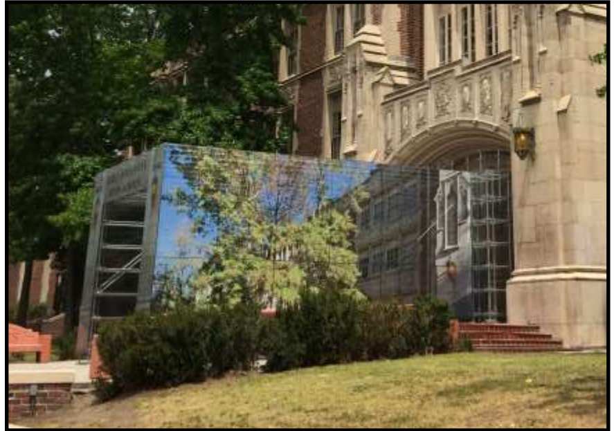
New scaffolding graces the front of John Marshall High School
