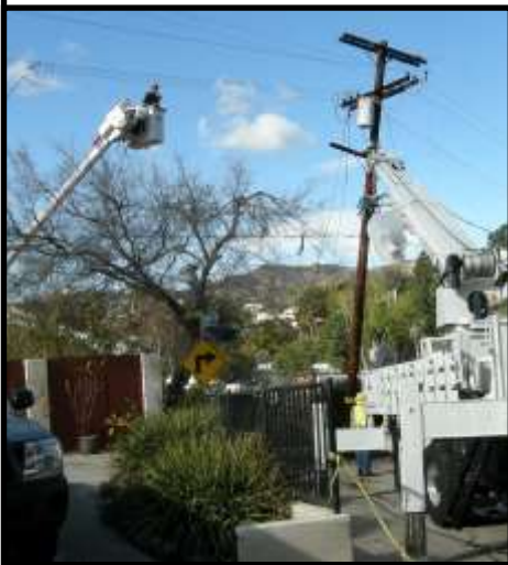
DWP Crew Uprights Downed Pole
