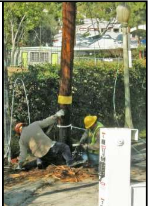
Workers Set Pole in Ground
