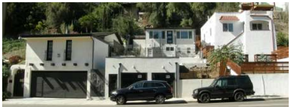
2205-2211 Hyperion after restoration of the three homes
