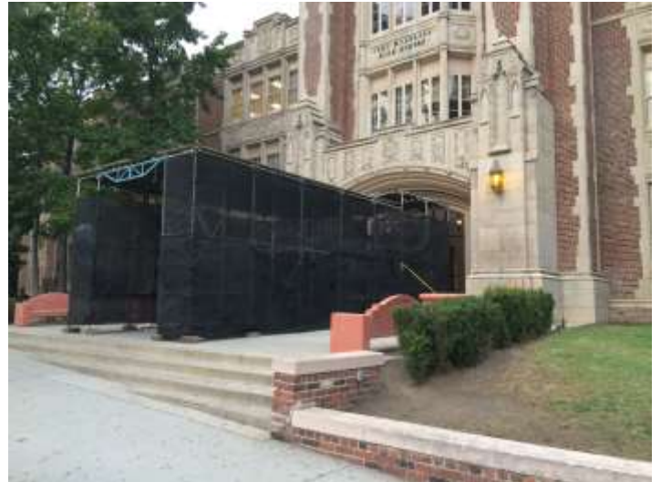
Scaffolding in front of Marshall High (photo by Charley Mims)
