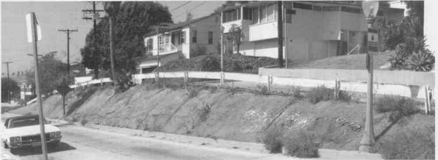
Median before asphalt was removed
