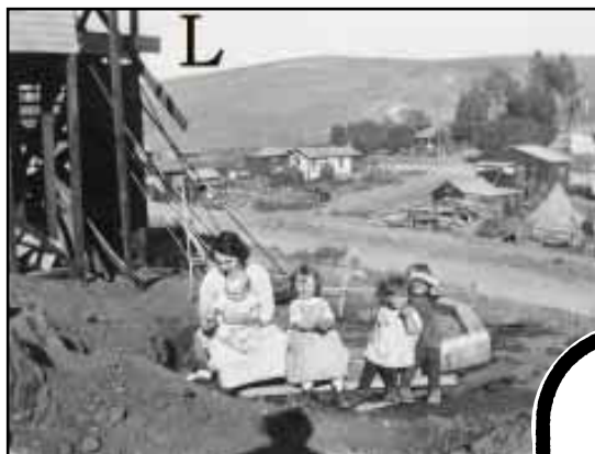
Corner of Hyperion & Lyric, 1922. Taken from beside Young family home at 3914 Sunset Dr. under construction.
