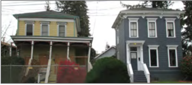
THE HOUSE ON THE LEFT WAS NOT RETROFITTED AND SLID OFF ITS FOUNDATION AFTER THE 2014 NAPA EARTHQUAKE. THE HOUSE ON THE RIGHT, WHICH HAD COMPLETED A SEISMIC RETROFIT, WITHSTOOD THE SHAKING.
