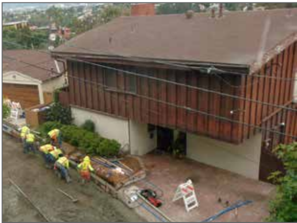
BUREAU OF STREET SERVICES CREW PLACING NEW CONCRETE 📷: BILL MOORE
