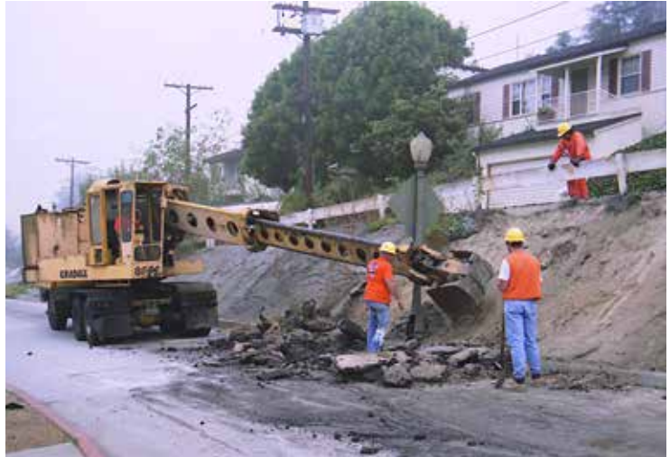
REMOVING CONCRETE FROM THE SLOPE, 1995
