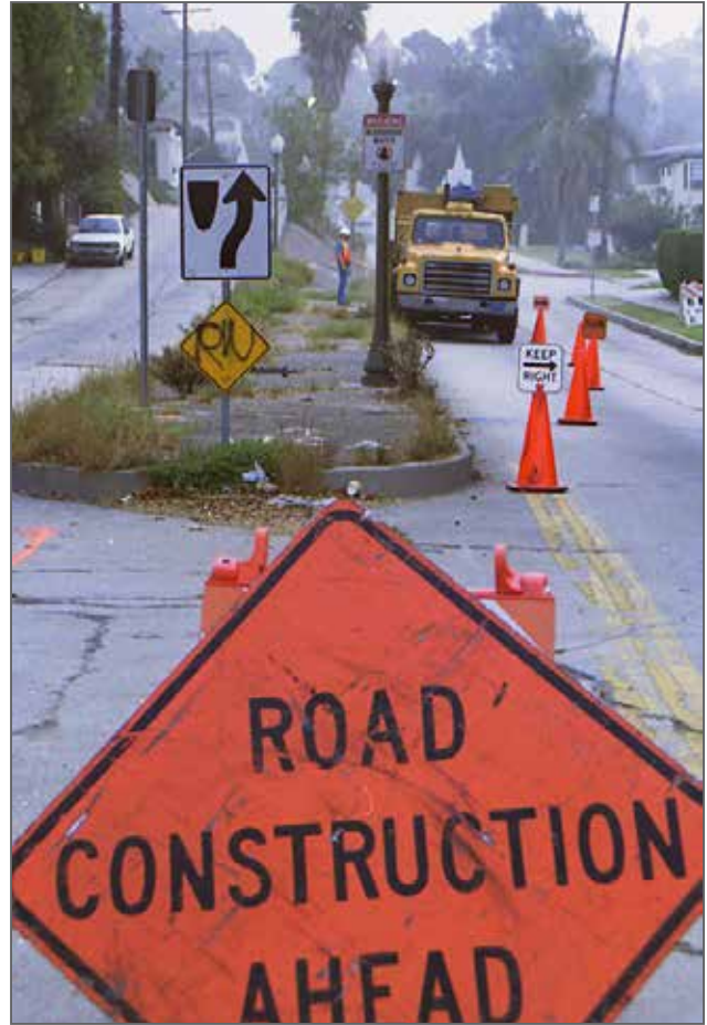
PREPARING FOR DEMOLITION, 1995
