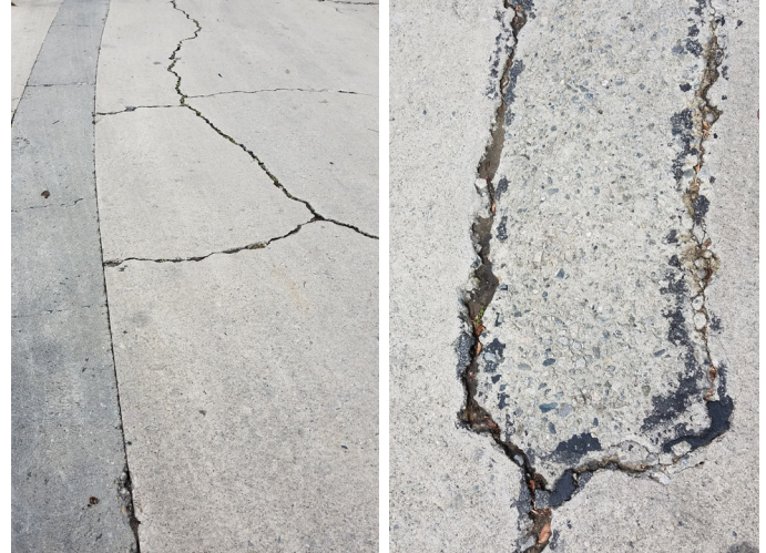
Left: Sawcut utility trench repair. Right: Old broken edged utility trench repair. Photos by Elizabeth Richardson.
