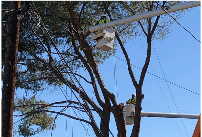
LADWP crew cut branches off the crown of the tree before removing the trunk. Photo courtesy Elizabeth Richardson.
