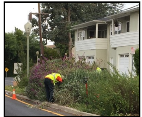
Cleaning up the median
