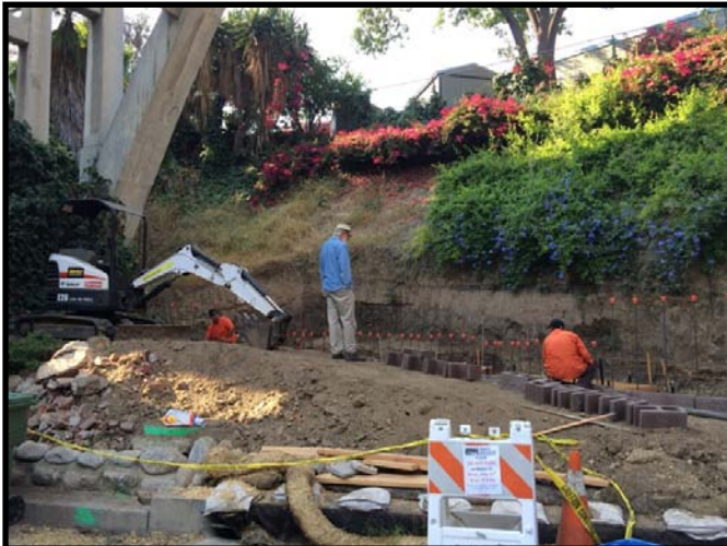
Charley Mims “inspects” progress for retaining wall.
